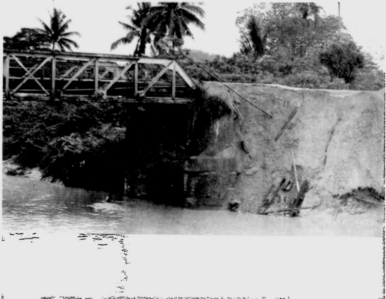
Danger of collapse...a slice of the river embankment by the old steel bridge in the former West Country Estate has been eroded away.
