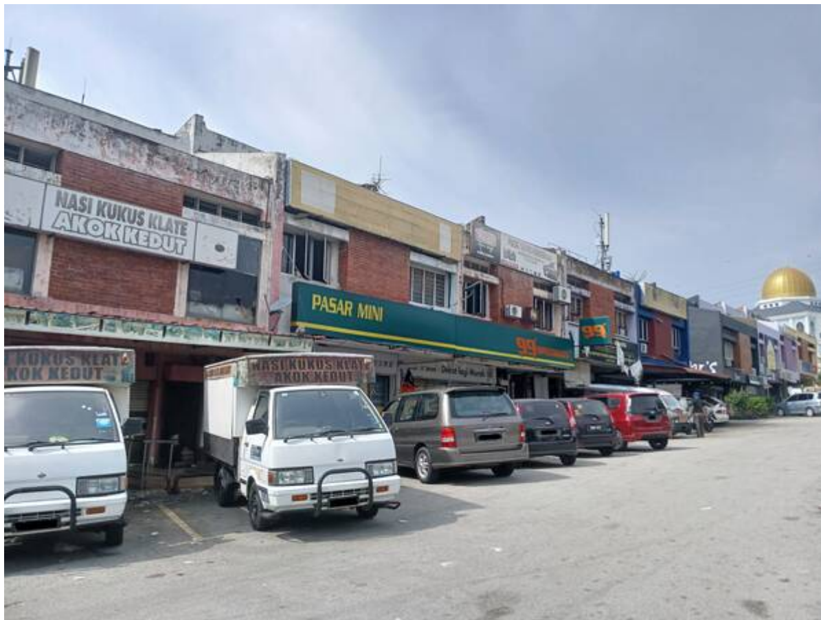
No. 4, Jalan 1/4 (99 Speedmart) (Gambar: Sazli Shahrir, 2025).
