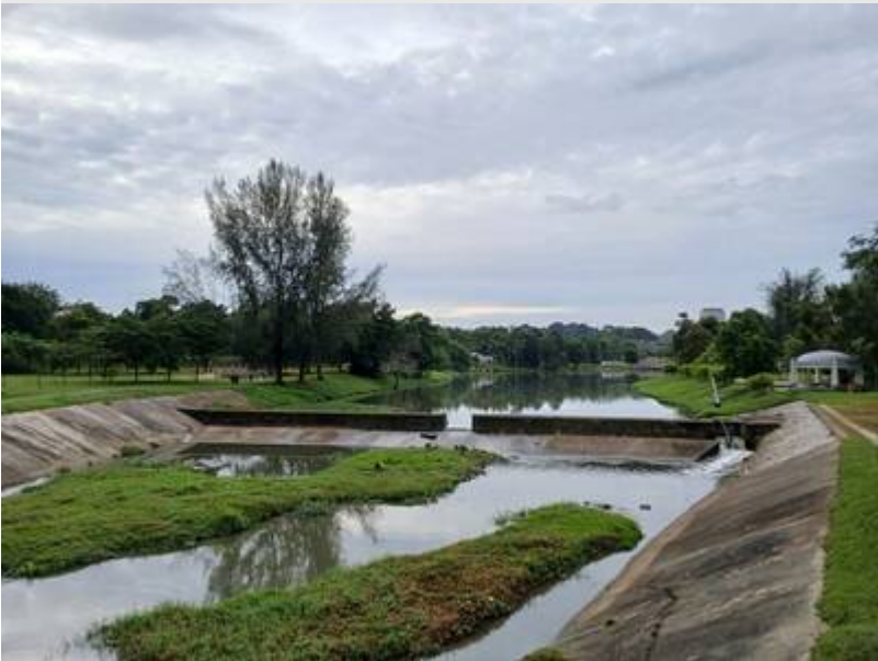
Kiri: Tasik yang hampir siap dibina. Gambar mungkin diambil di jambatan Sungai Air Hitam, Persiaran Bangi, menghadap ke selatan: “Work in progress ... to level the river bed of Sungai Air Hitam and developed it into a lake garden.”
