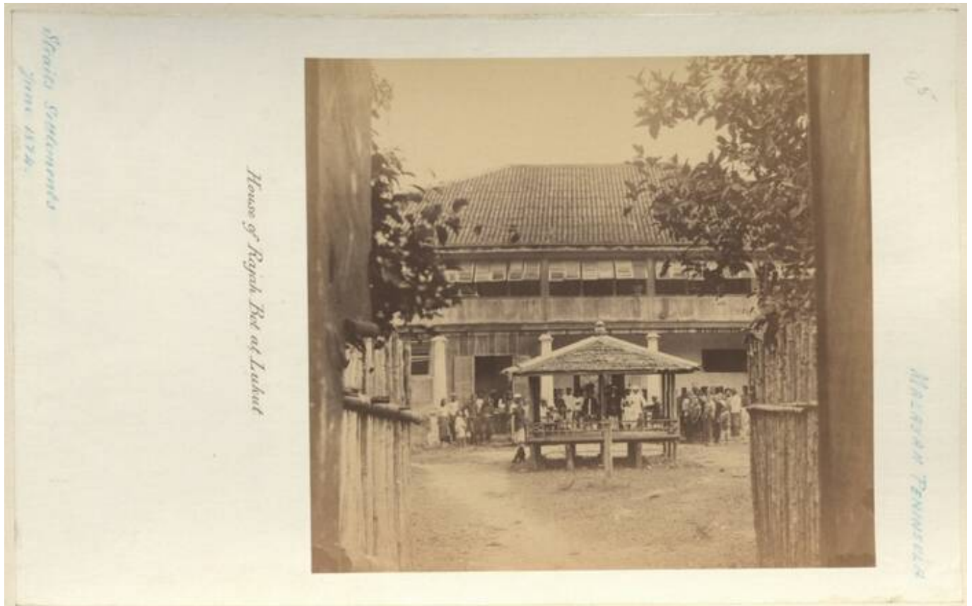
"House of Rajah Bot at Lukut. Straits Settlements June 1874." (The National Archives UK, June 1874:
