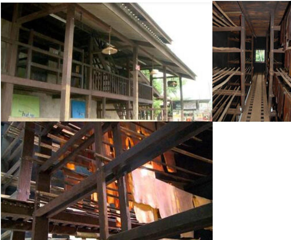
Setelah dibaikpulih. Kiri: “Racks of smoking room for rubber sheets hung on bamboo poles (2007)” . Tengah: “Racks of smoking room for rubber sheets hung on bamboo poles (2007)” . Kanan: “The timber in the Smokehouse was found intact and well preserved. Years of smoking the rubber, and by association the timber, had not only preserved the wood but also hardened it further (2010)” .
