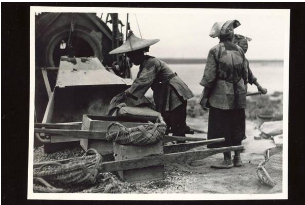
"Samsui' women working at a construction yard, 1938-1938. Collection of National Museum of Singapore."
