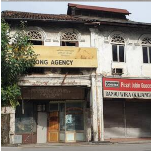
Kedai terawal dibina pada tahun 1896: No.1 Jalan Besar: “In 1896, 40 shop houses were built in Section 1 which covered Main Street, Tukang Street, Jln. Tengah and Mendaling Street. This shop house which is no.1 at Main Street and the one beside could be of earliest batch or built within the decade. This corner lot was said to be acquired and demolished to give way for road broadening. Or, should it be conserved and restored and repurposed to mark the history of establishment of Kajang Town?”
