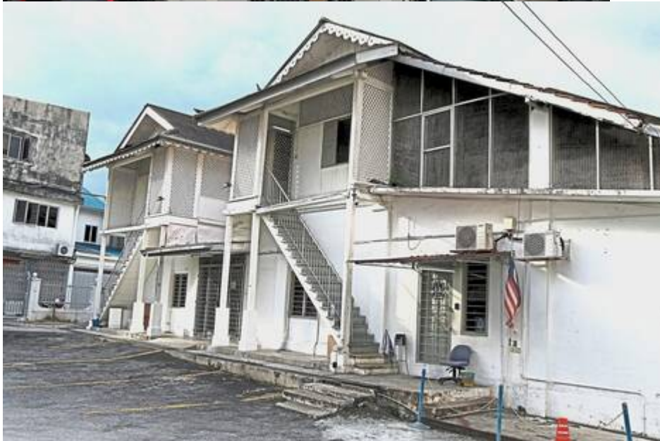
Kiri: “Located on Jalan Tengah, the building was built before WWII, and started operations in 1914. It was made with cengal and meranti wood, and has undergone renovation over the years. The design is a mix of traditional Malay classic and colonial European style. The building is a post office till today.” (Hanna Hussein @ New Straits Times, December 19, 2019:
