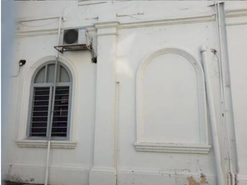
“Kajang Post Office is the only building with adaptive Tudor domestic style in town. The upper floor is timber based Malay vernacular traditional design with wooden louvre & large windows. The two stairs at rear side add to its beauty. Lower floor has relatively large pillars and arched windows built with bricks. As told by the senior officer, it was built in c.1910s, the shaping years of Kajang township. This architectural jewel has now been included as one of the seven heritage sites in the Kajang Heritage
