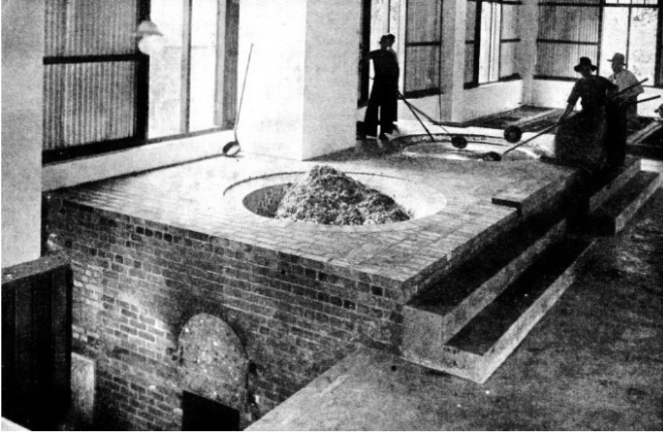
REFINING PANS in the Chinese smelting plant at Kuala Lumpur, Malaya. The tin is smelted in these pans and the slag, which rises to the surface, is skimmed off with ladles. The skimmings can be seen in the pan in the foreground. This is the only Chinese smelter left in Malaya, the rest of the tin being smelted by two European companies.
