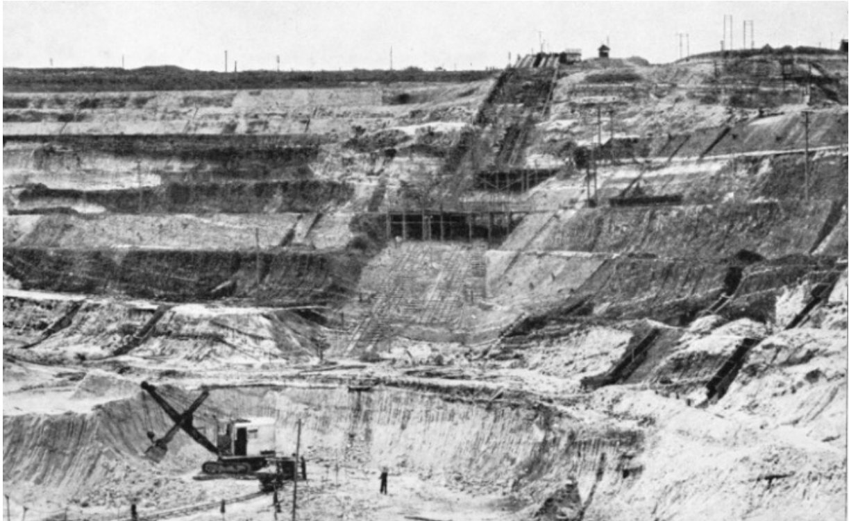
THE LONG INCLINE up which excavated material is hauled to the puddlers on the surface. The photograph shows the Hong Fatt Mine , one of the largest open cast mines in the Federated Malay States. The mine is 3,700 feet long, 1,600 feet wide and nearly 300 feet deep.
