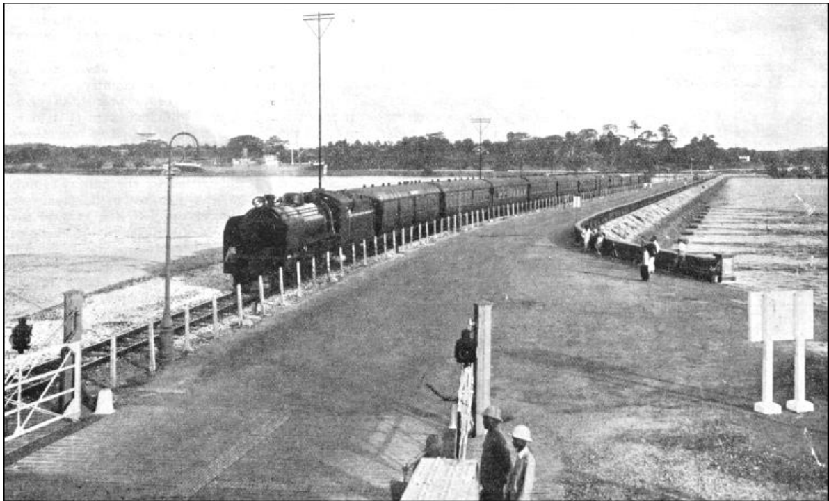
ACROSS THE JOHORE CAUSEWAY. A mail train of the Federated Malay States Railways on its journey from Singapore to Kuala Lumpur, a distance of 264-1/4 miles. The causeway is 60 ft. wide, has a length of 3,465 ft., and connects the mainland with the island of Singapore.
