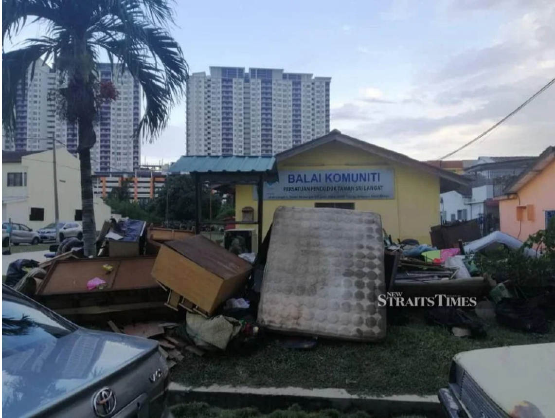
A community hall in Taman Sri Langat in Jalan Reko becomes a dumping ground.
