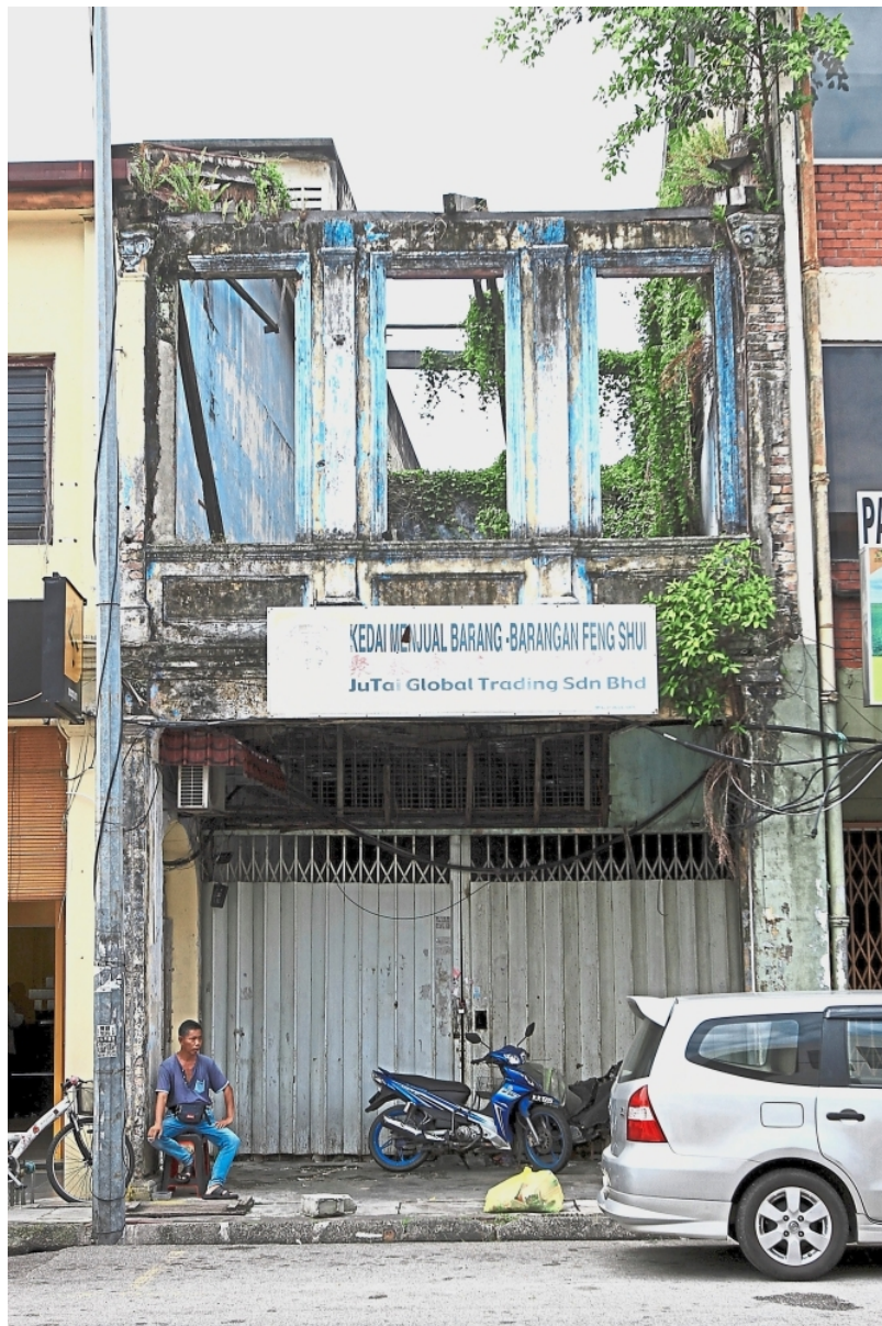
The shophouses in Pekan Ampang, many of which have reached 100 years old, makes them eligible as heritage, are either in bad weathered conditions or defaced with convenient renovations.
