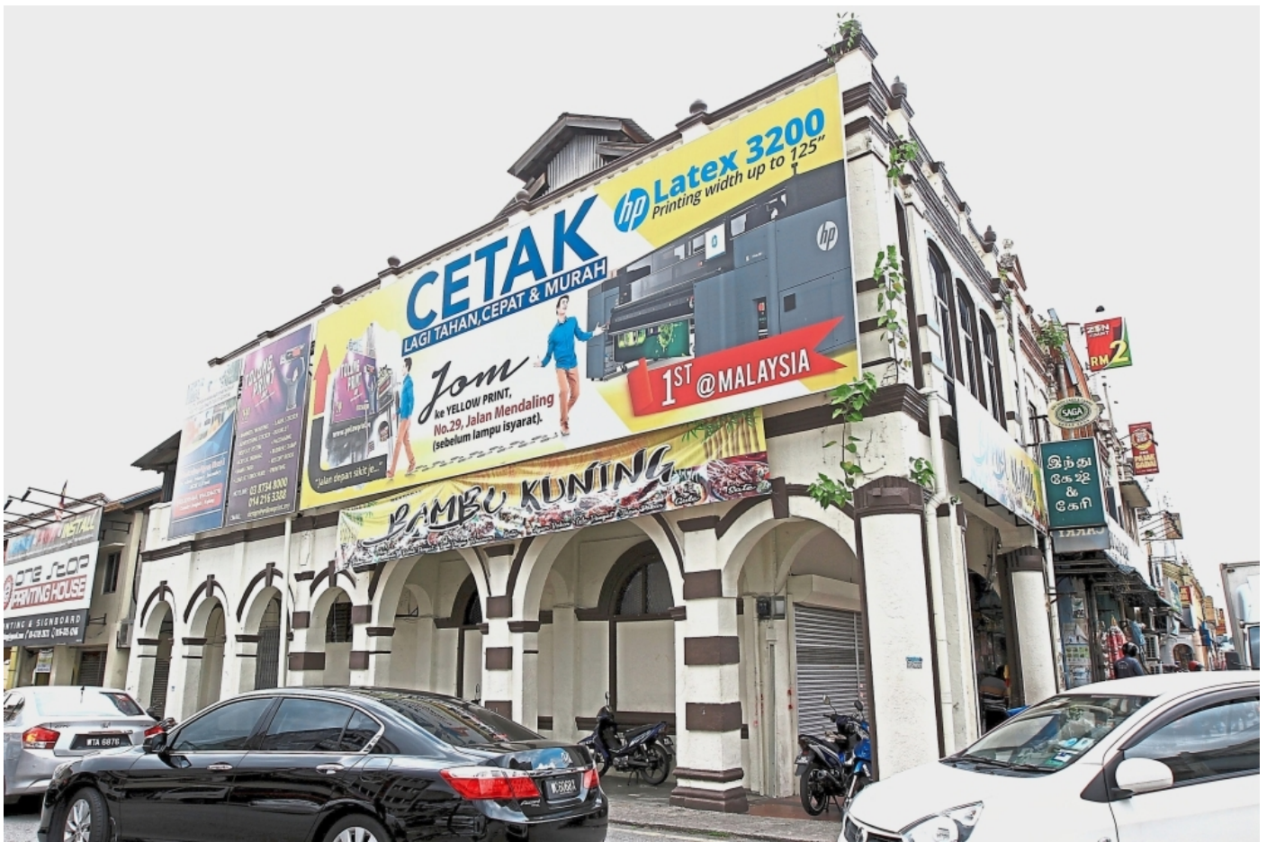
The unique architecture with embossed words on the wall of this century-old shophouse in Kajang town is covered by billboards. — Photos: LOW LAY PHON/The Star
